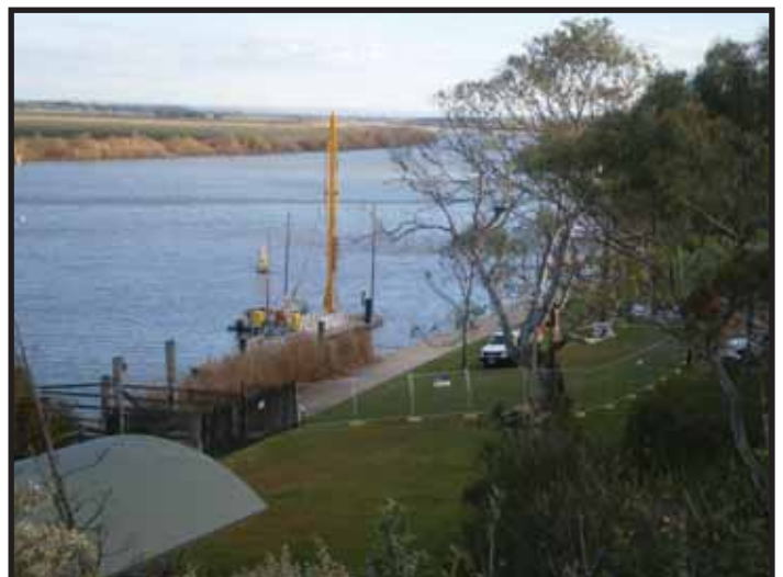
ABOVE: The upgrade at Dickson Reserve.
