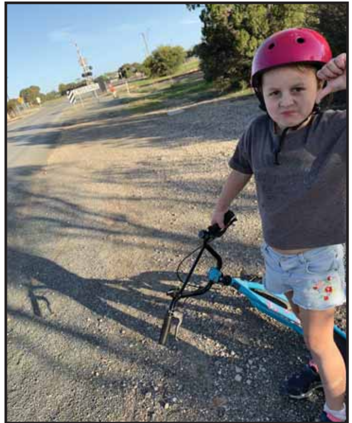
ABOVE: Hailee of Tailem Bend disappointed with the cracks on the footpath.
